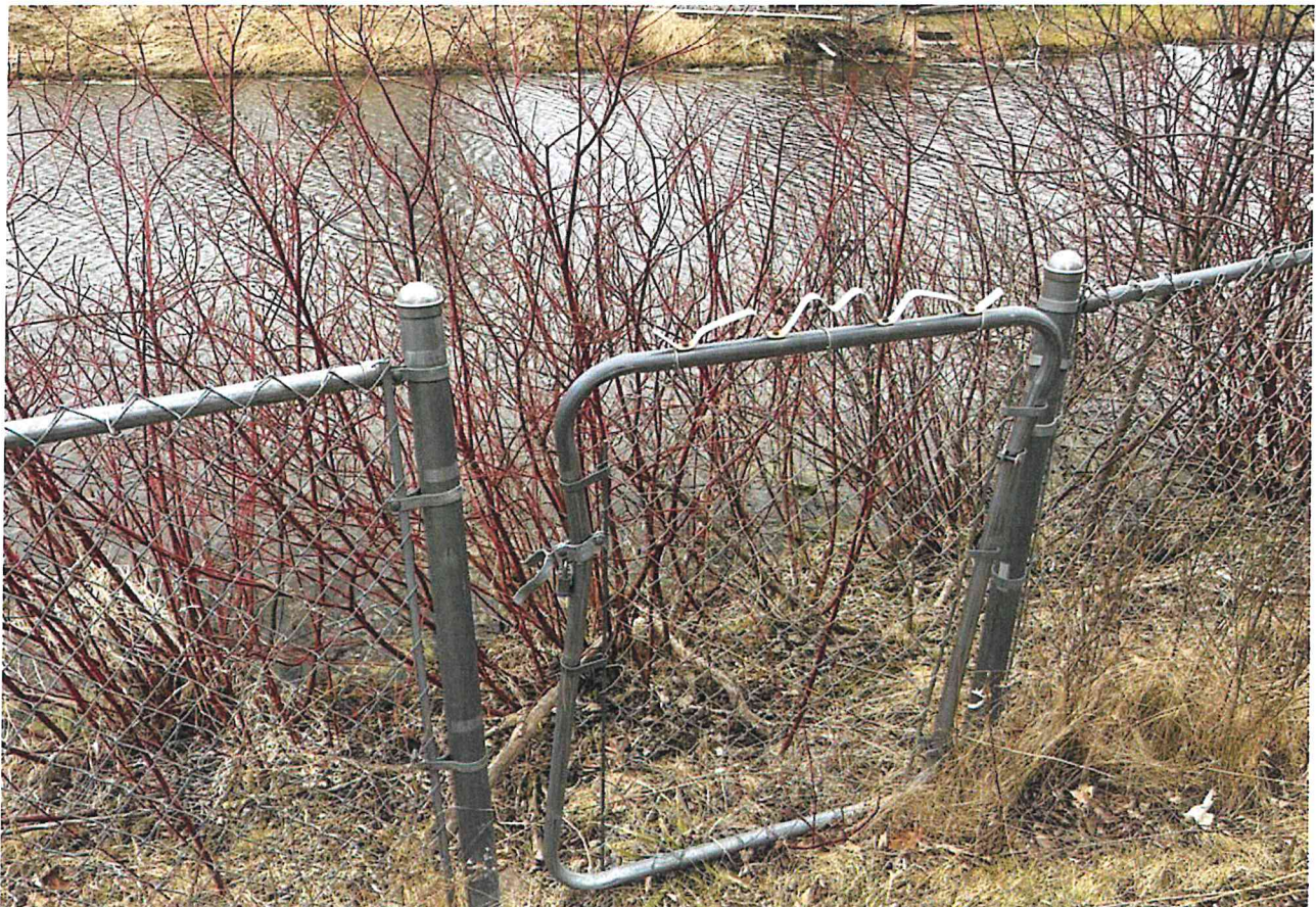
Damaged fence gate
