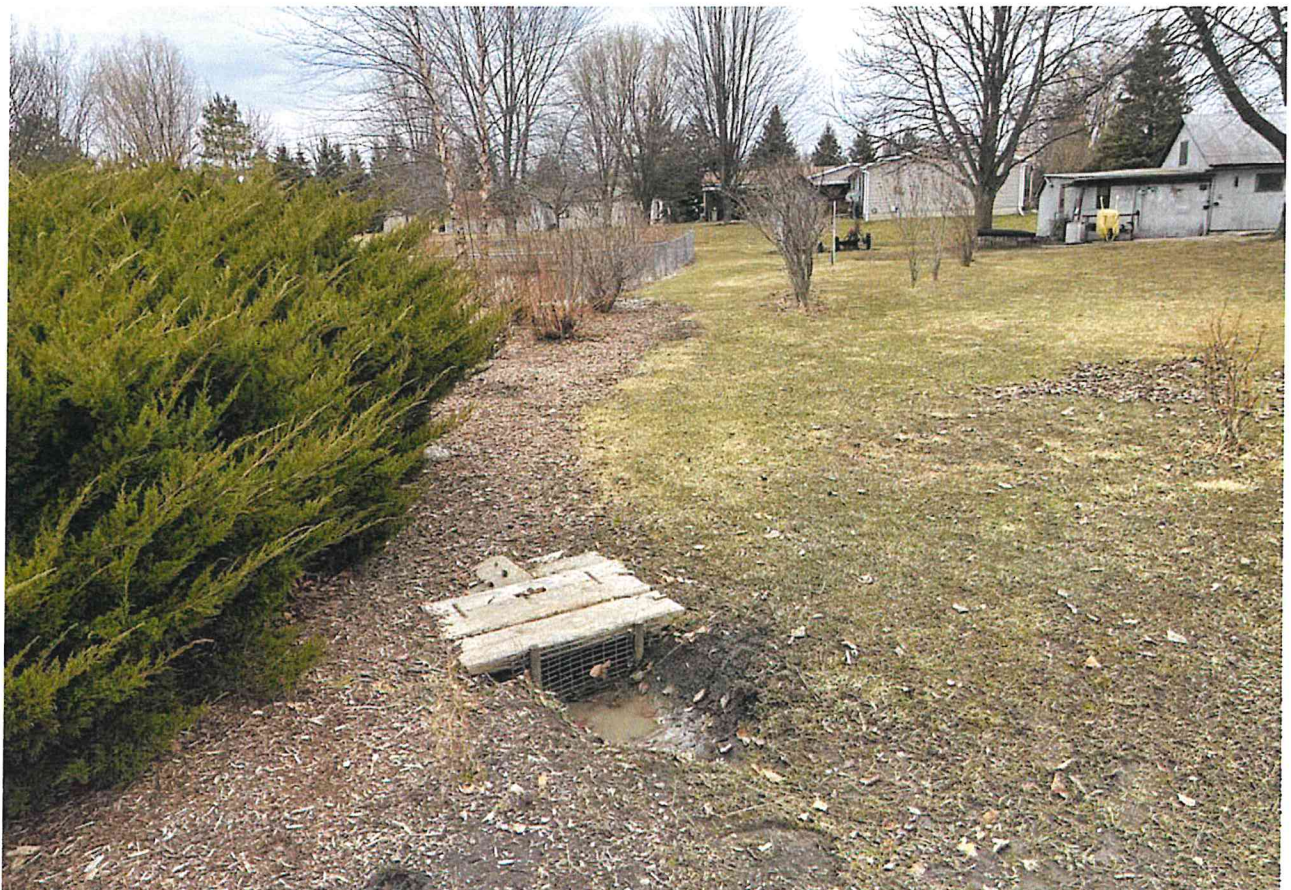
Storm water inlet to adjacent non-subdivision parcel
