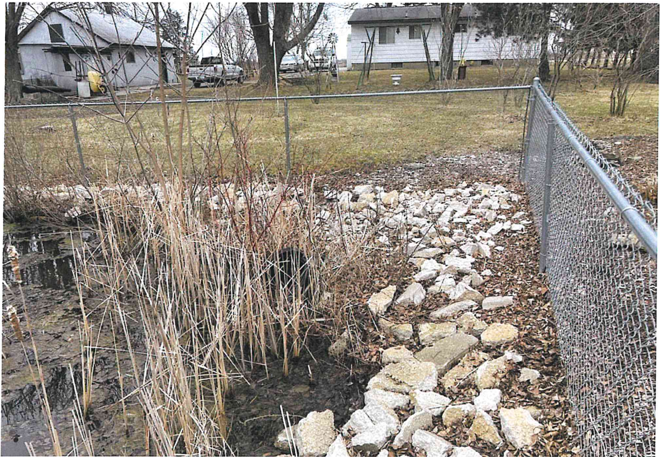
Detention pond outlet
