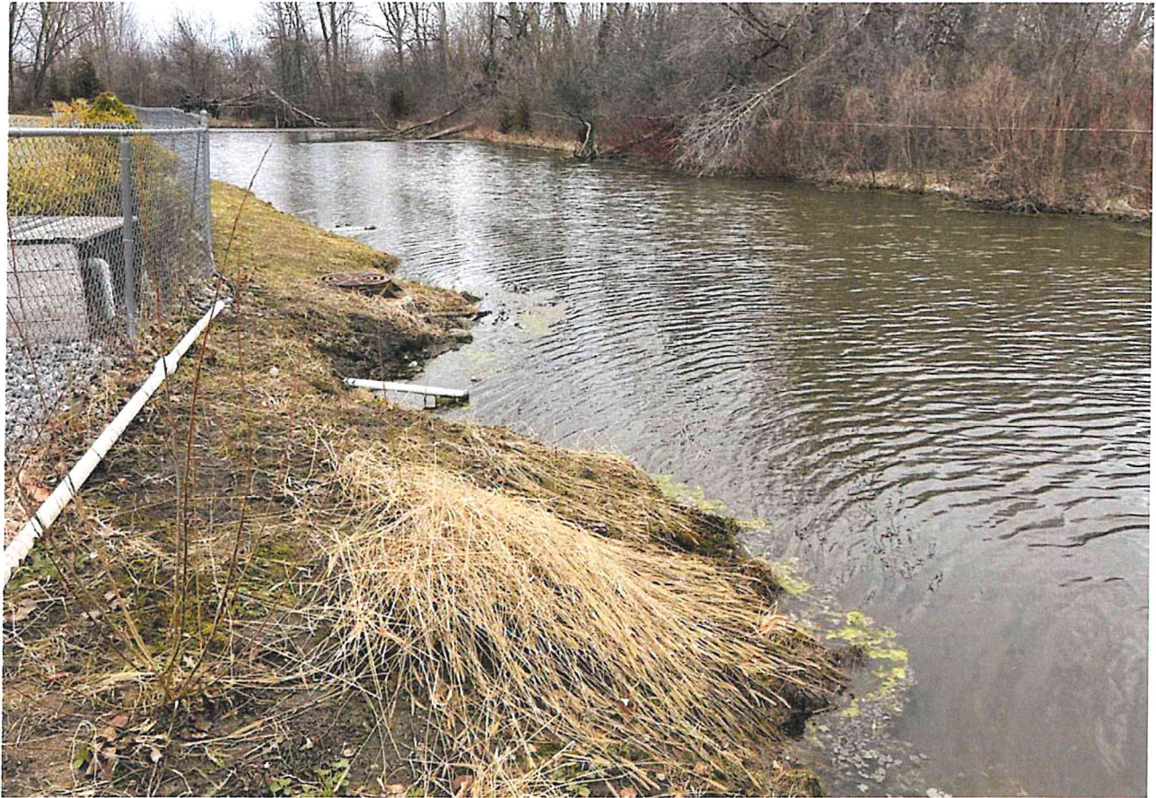
Pump house on south side of detention pond
